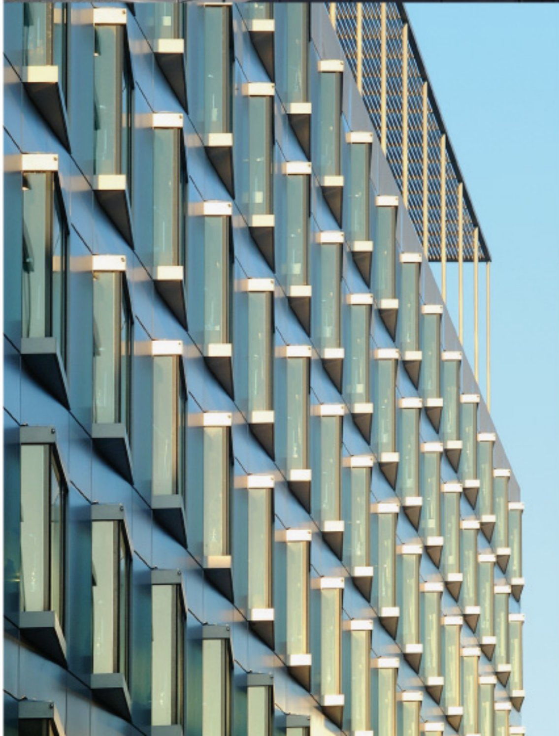
above: Eastern side below: Facade detail right: Ground plans ground floor, 1st floor and longitudinal section
